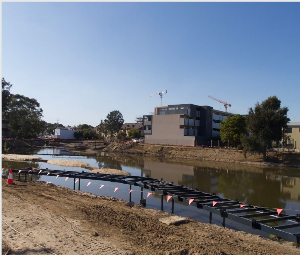
Figure 27 Boardwalk under construction (Babb 2020)
