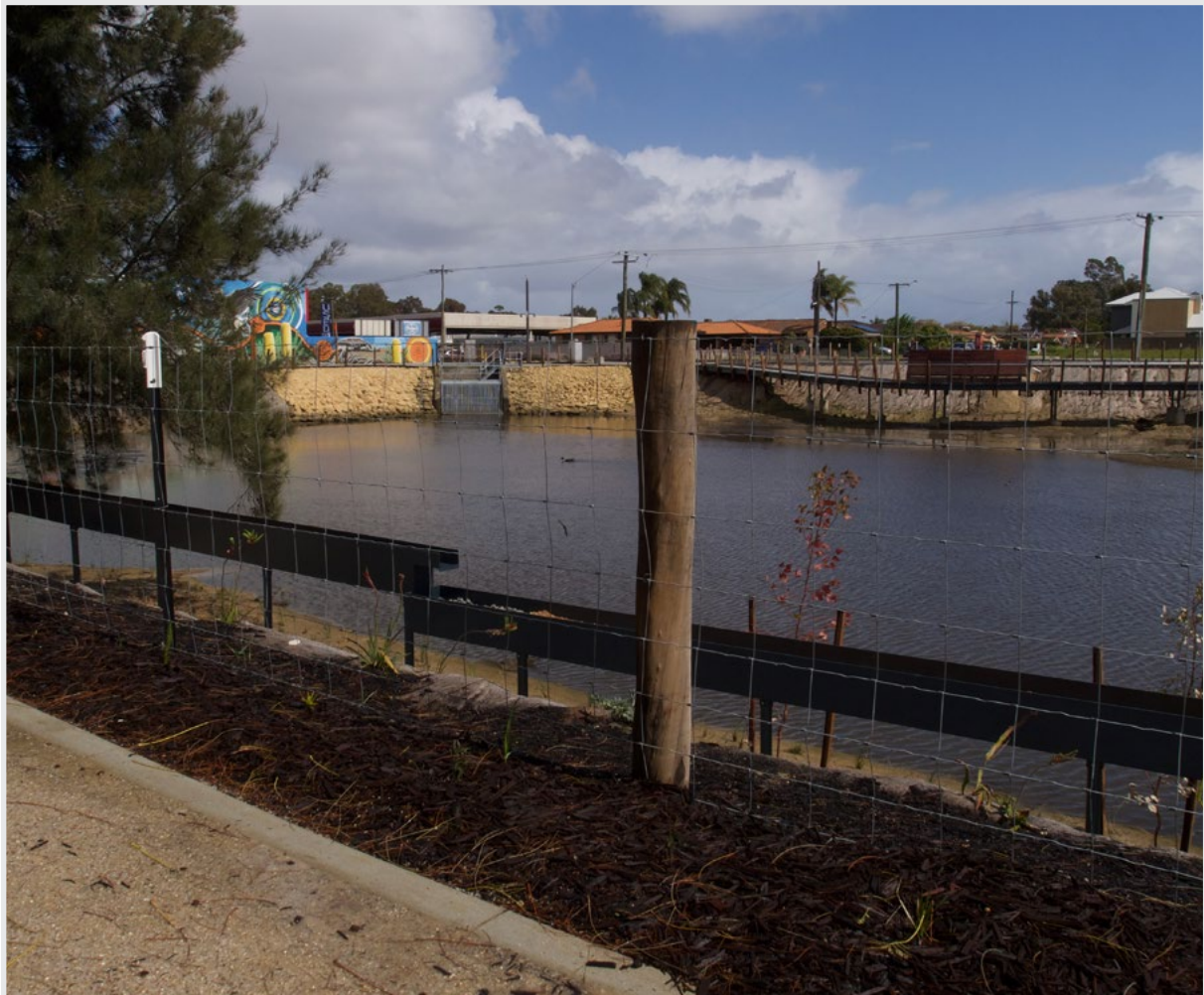
Figure 59 Simple jarrah and wire fencing around park perimeter (Babb 2020)
